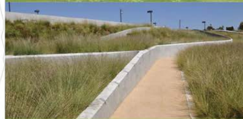
Terraced Retaining Walls
