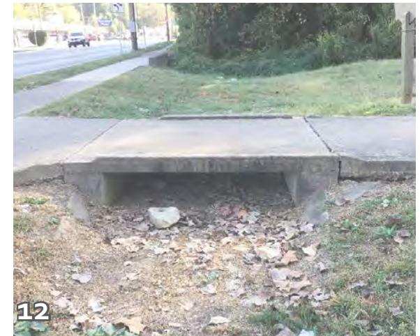
MASONRY BRIDGE - concrete, spans ditch directing runoff to culvert (1979)
